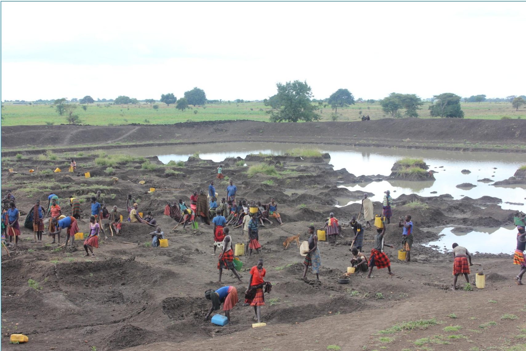
Karamojong at work – digging (to expand) a valley dam at Lokitelarechek in Kotido district as a way to “catch” the little rain water while it lasts. Wendy Daphne Kasujja, 2014
